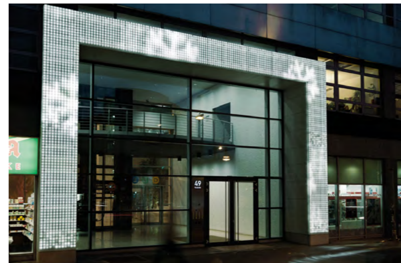
Customers of this office complex are enthusiastic about the animated snowflakes visible on its façade.
