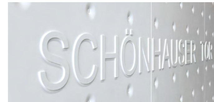
Effectively animated outside, inside a clear design of dots and letters milled out by using the CNC technology.
