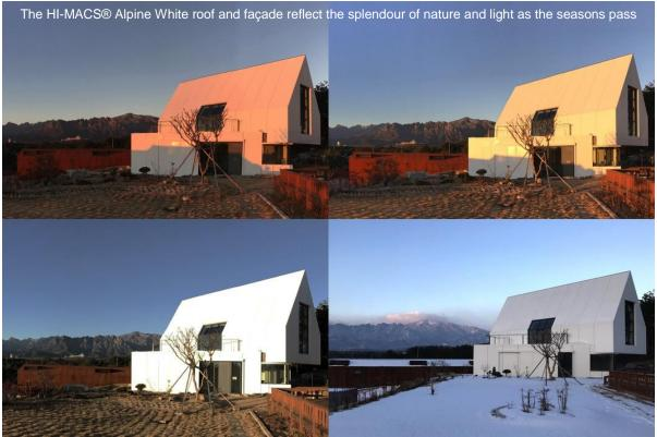
According to Woojin Lim, "The decision to use HI-MACS® to create the façade was obvious. One of the main causes of alterations to a façade is rainwater run-off. With HI-MACS®, the seamless assembly provides a solution to the vertical grooves in other materials that make the structure permeable and hasten the façade's deterioration over time".
