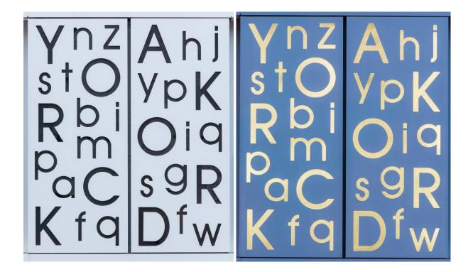
For the façade's architectural design, the letters were milled into the HI-MACS® surface using CNC technology, and each one has a unique design. The structure is backlit for a more dramatic effect, and its sides are slightly contoured with an LED light to soften the letters that make up the poems.
