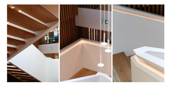
Further enhancing the wood, the railings installed all along the path of this atrium structure – with the exception of the landings – are cladded with 12-mm bonded, seamless HI-MACS® Alpine White panels, on top of a metal structure with a slightly beveled lip.
