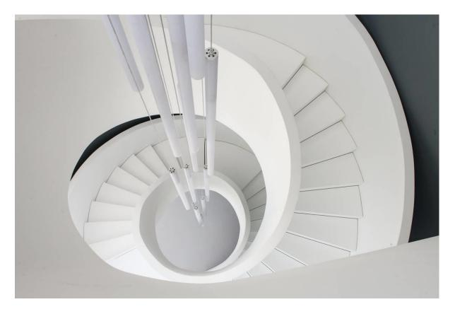
In order to accommodate the LED lights, the steps had to be milled having first had an extra piece of material added, to increase the thickness of the step. Finally, thanks to a skilful and innovative solution, the steps were made so as to fasten onto and be released from the structure by means of a magnet system which, by making everything easily removable, also makes it very practical to remove the electrical system in case of a fault.
